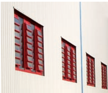
JET-SMOKEJET® surface ventilator installed in the facade for ventilation, SHEV-air intake and daylight
